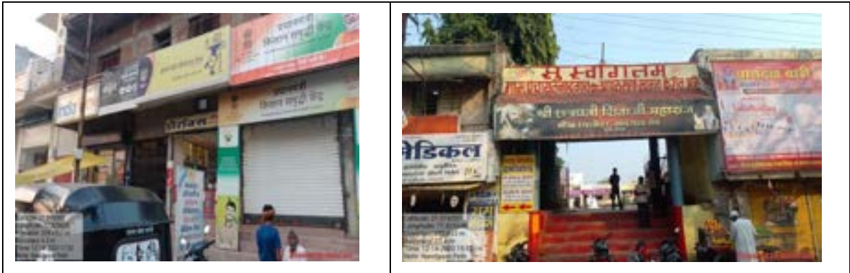
Market facility at Nandgaon Peth
